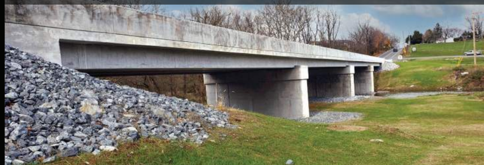
SR 1003-022 Design-Build Bridge Replacement over Little Swatara Creek, Lebanon, PA
