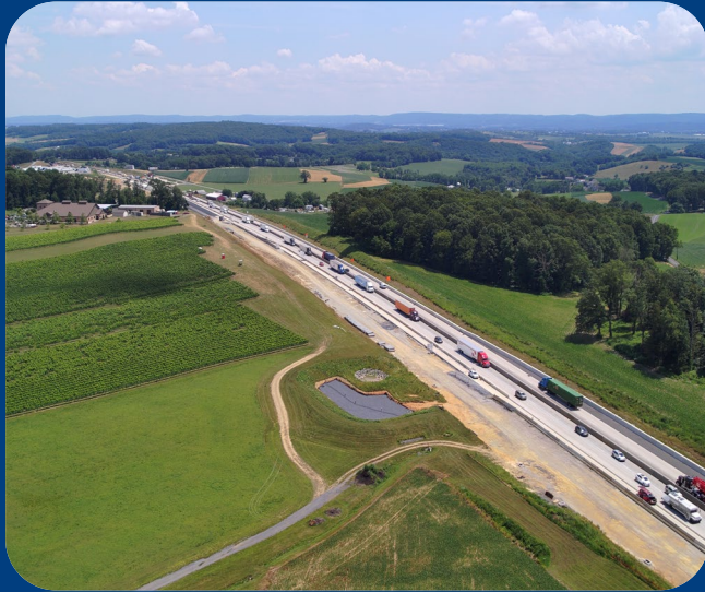
SR 78 Reconstruction and Widening
