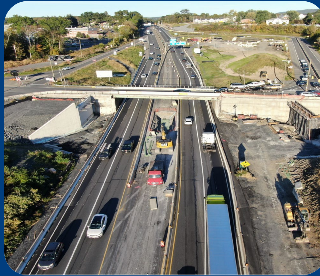
SR 80 Realignment and Bridge Replacement
