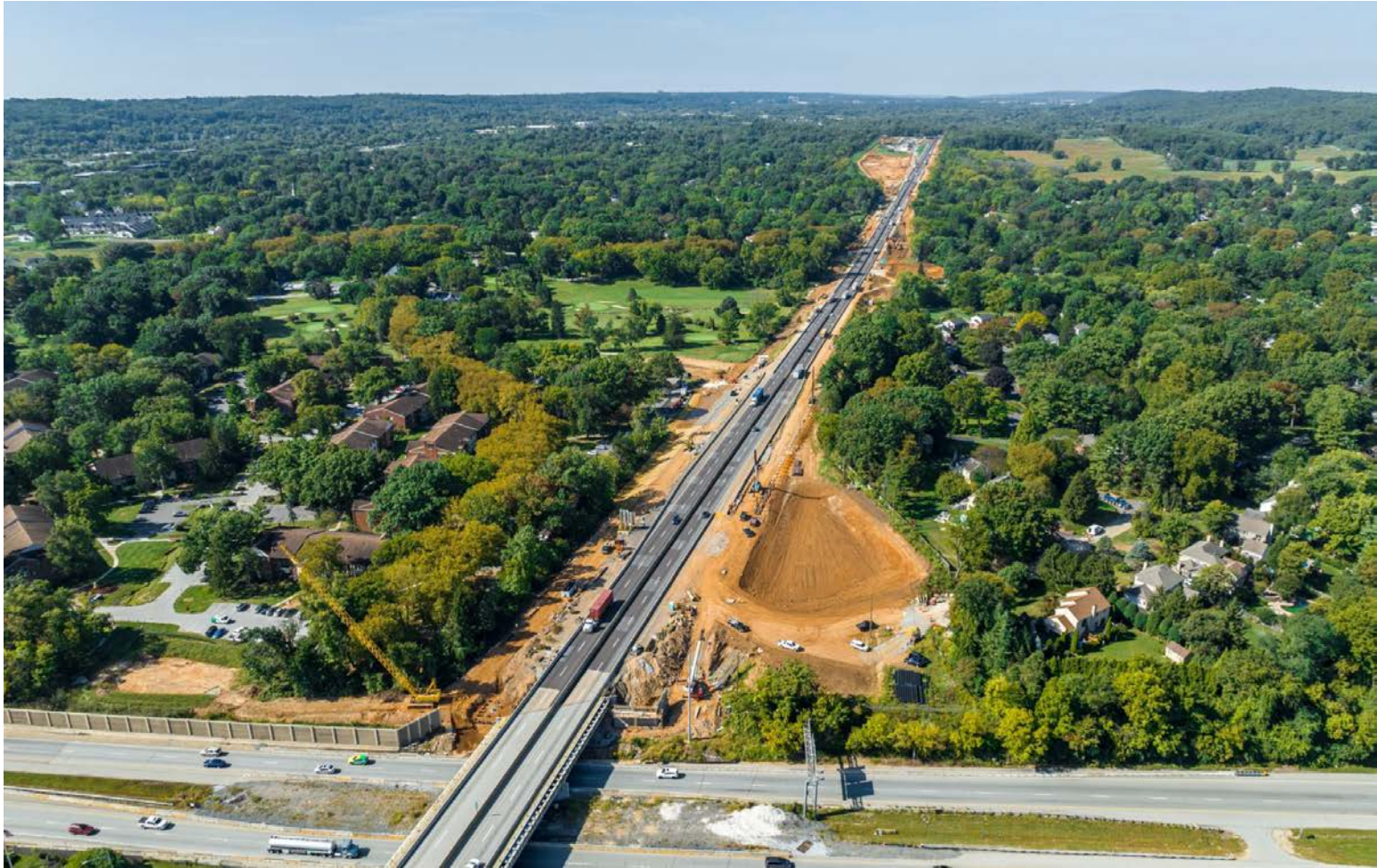
Stage 1A Looking West
