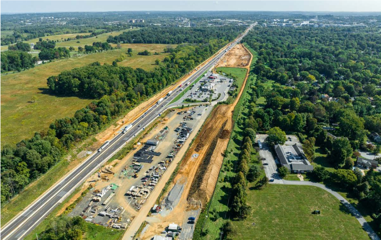
Stage 1A Looking East
