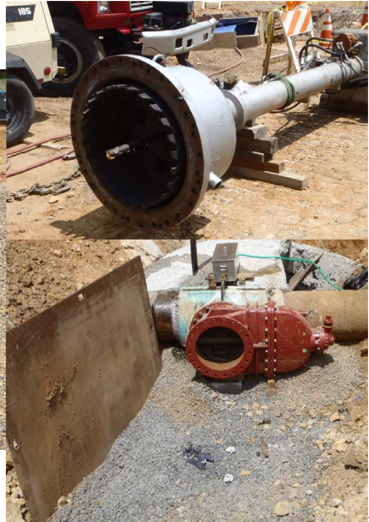
Jacking pit for installation of two 48-inch sleeves under US 422
