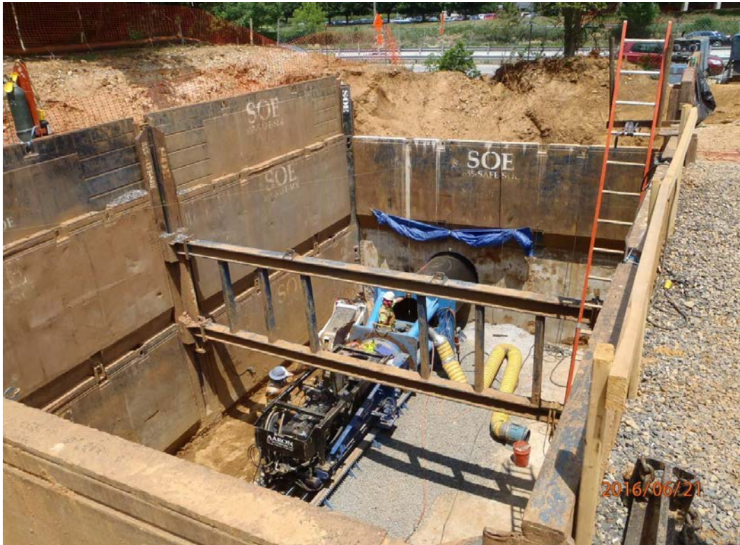
Jacking pit for installation of two 48-inch sleeves under US 422
