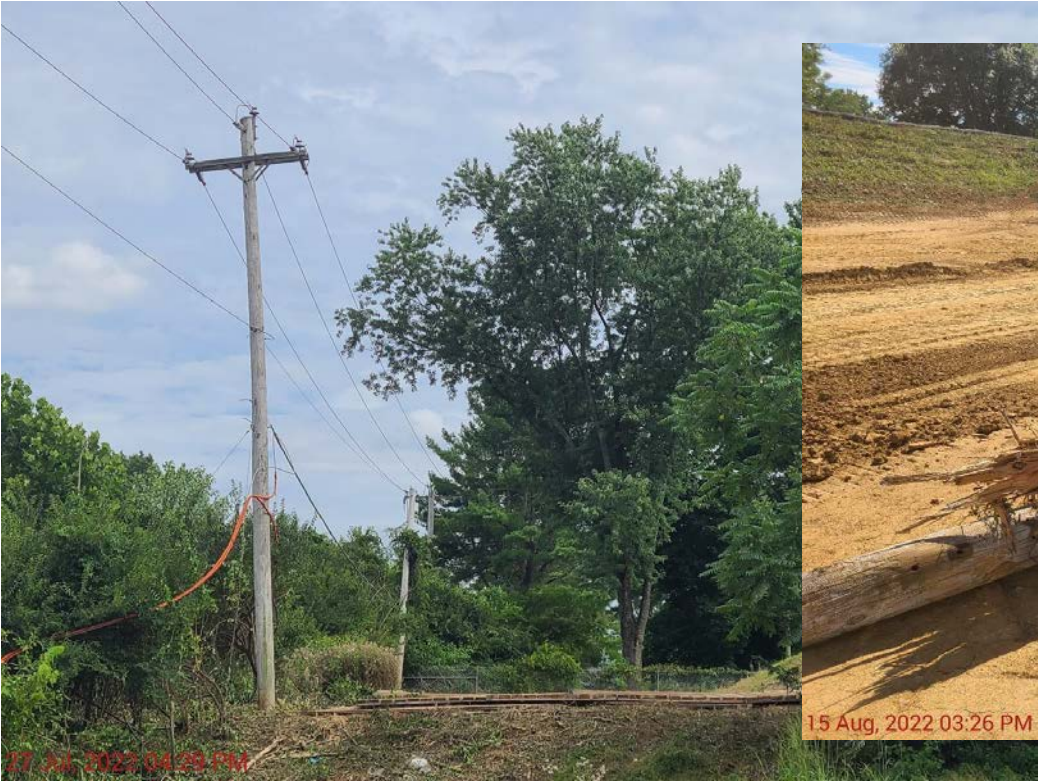
PECO Pole in Conflict with Excavation
