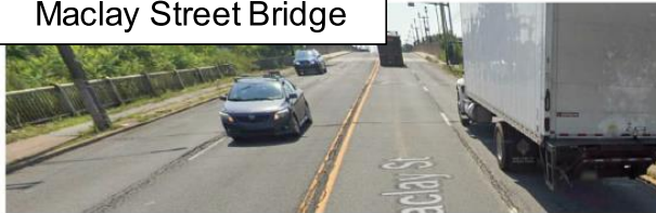
Existing 4-Lane Roadway
