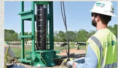
Remote Dynamic Pile Analysis
