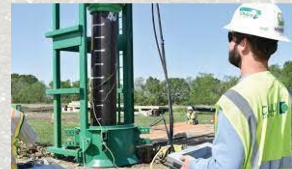
Remote Dynamic Pile Analysis
