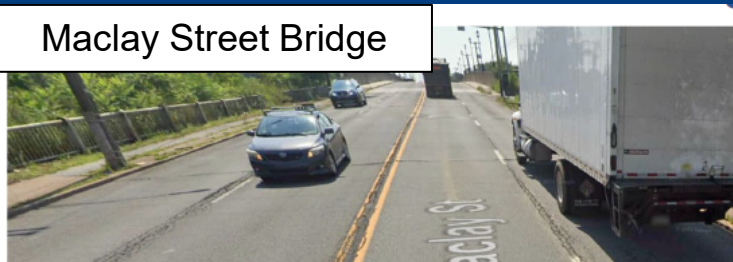
Existing 4-Lane Roadway
